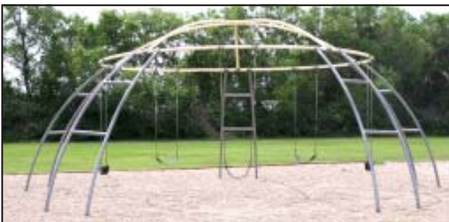
Round swing supports can present a problem of inadequate interior use zones.
