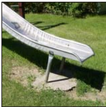
Exposed concrete footings under play equipment create a trip hazard.
